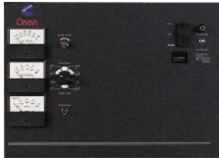
Figure 4-17. Two-Wire Control Interface Panel
