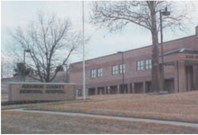
At Audubon County Memorial Hospital, paralleling load transfer equipment eliminates power surges during monthly testing.
