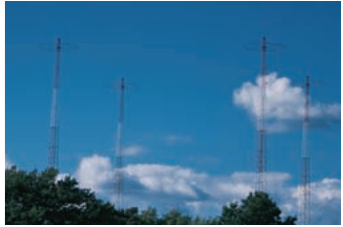
Nearly 300 Verizon Wireless remote cell sites are backed up by standby generators from Cummins Power Generation.
