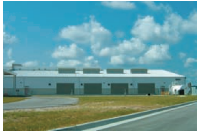
The standby power system is housed in a power building located one-half mile from the Phase-V facility.
