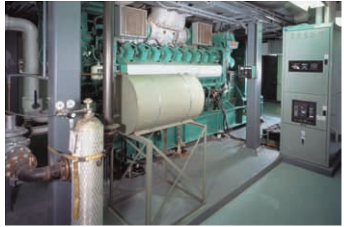
The PowerCommand QSV91G gas engine generator from Cummins Power Generation produces 1,250 kW and over 10 million Btu of heat per hour.
