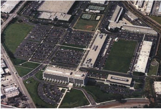
Waste heat from the generator is used to run a 250-ton absorption chiller for the campus's air conditioning system.
