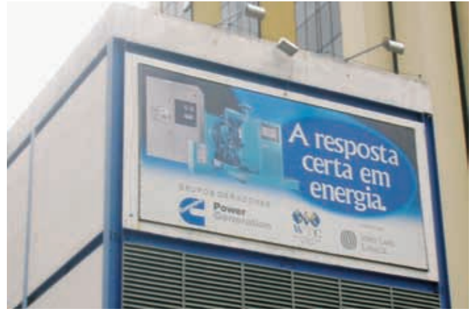
This three-story power building that houses generator sets is designed to blend in with the rest of the complex.
