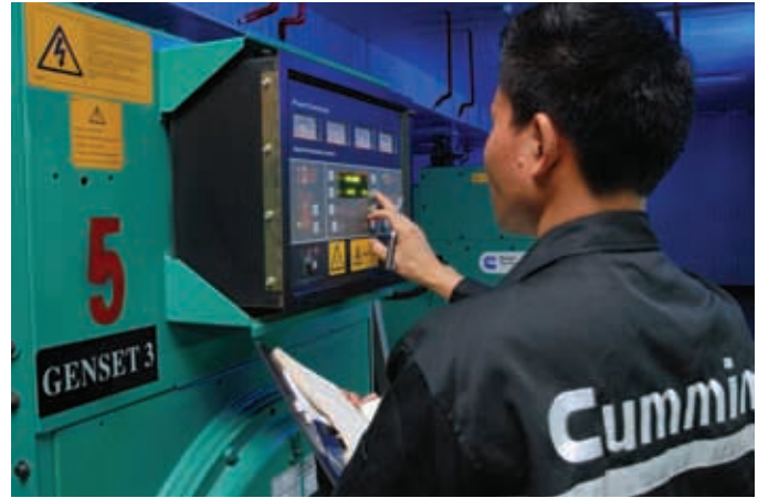
PowerCommand controls on each generator set are easy to use and provide real-time system status as well as system integration and remote control functions.
