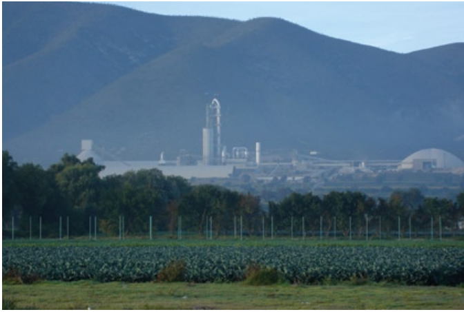
The new Cementos Cruz Azul plant at Palmar del Bravo, Puebla, Mexico, will produce 3,000 tons of cement per day when in full production.
