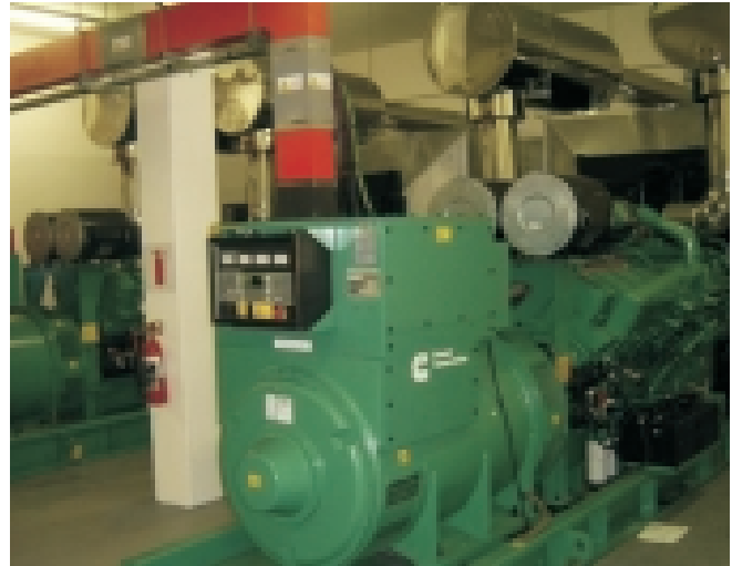
Installation of two C1400 D5 generator sets
