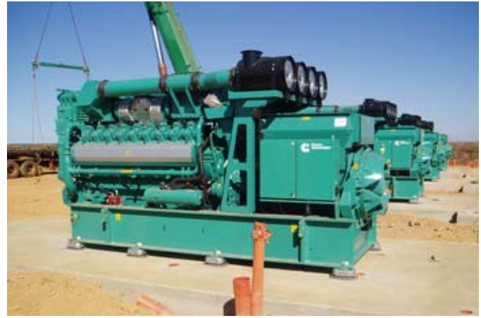
The QSV911 gas gensets are powered by lean-burn, spark ignited Cummins gas engines — 91-liter, v18 units with turbo-charging and after-cooling.
