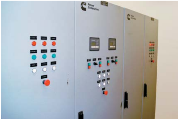
The DMC1000 controllers provide supervisory and power transfer functions with PowerCommand digital paralleling controls.
