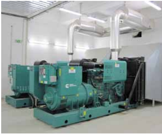
Installation of C900 D5 generator set
