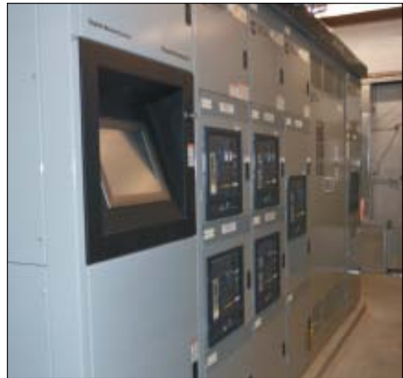
The PowerCommand DCM 200 digital master control contains the system operator interface and controls system-level functions including load add and load shed sequencing, as well as load demand.
