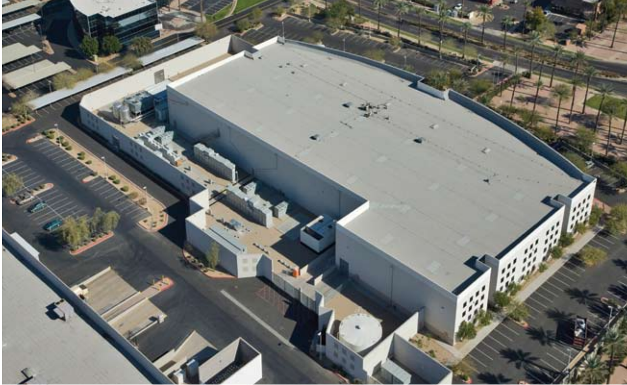
The 160,000 square-foot data center is equipped with redundant, reliable systems in a disaster-proof environment.
