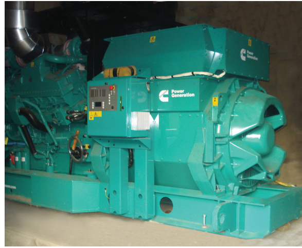
20-year-old generators have been replaced by new Cummins equipment
