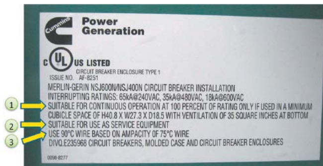
Figure 2 - (1) The 100% CB assembly must be labeled by the manufacturer as being 100% rated; (2) Equipment has to bear the marking "suitable for use as service equipment"; (3) Use 90°C rated conductors but size based on ampacity of 75°C.
